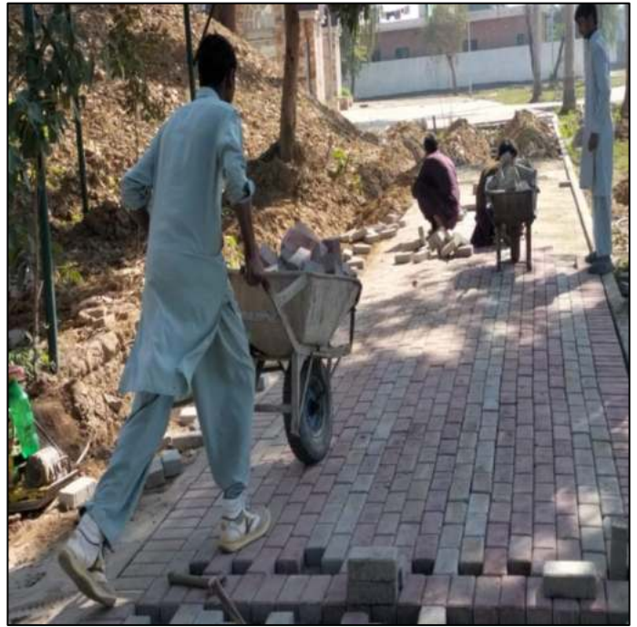
Picture 6: Tuff paver fixing on walkway @ Gulshan-e-Iqbal Park
