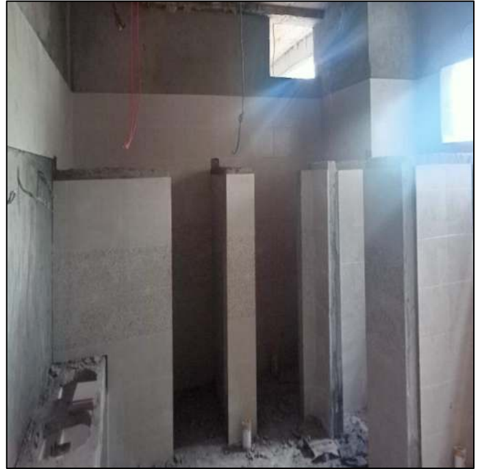
Picture 47: Porcelain Tile work in washroom
