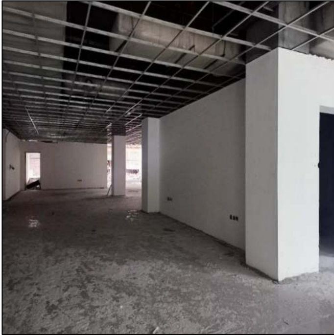
Picture 46: Paint work on walls of Ground floor
