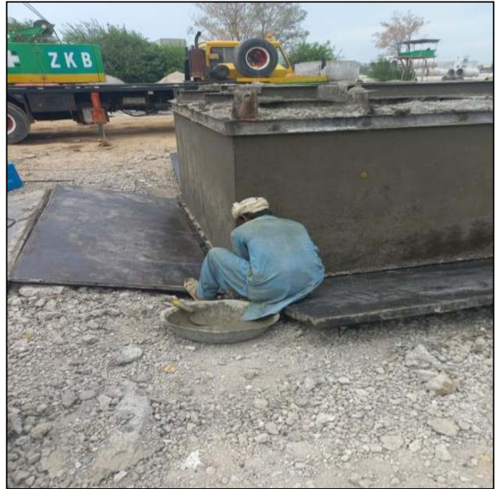
Picture 34: Lot-02: Conduit Formwork Opening in Progress @ Contractor Camp
