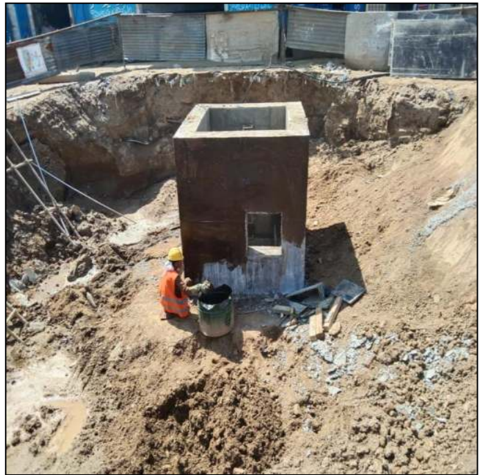
Picture 26: Lot-02: Manhole 50 Bitumen Coating in Progress at Marala Road
