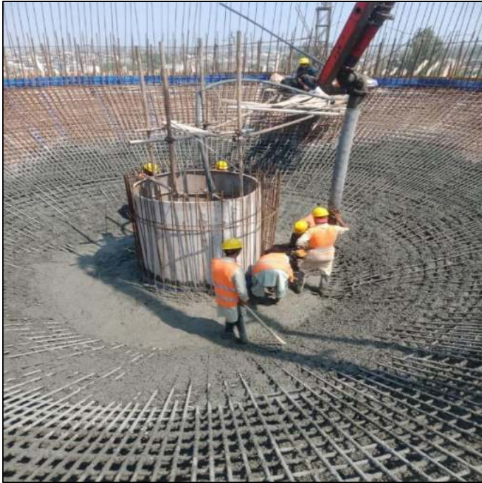
Picture 9: : Bowl Concrete Pouring of OHR T5
