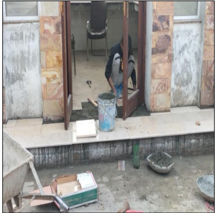
Picture 8: Fixing of China Verona in Kiosk of Gulshan-e-Iqbal Park
