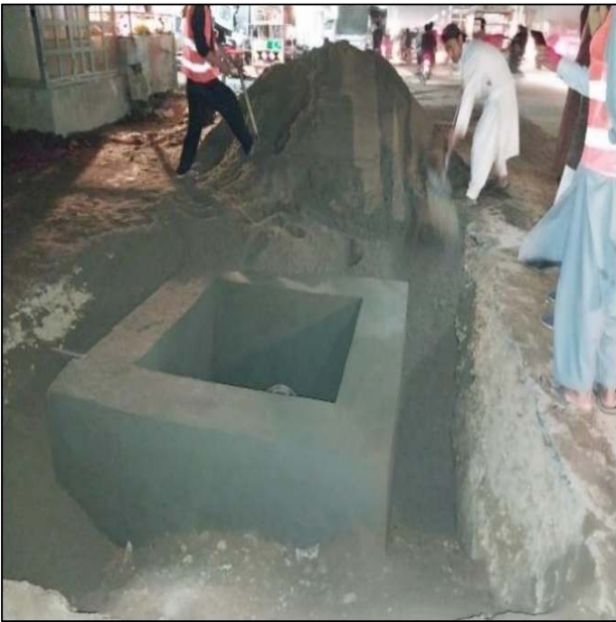
Picture 41: Isolation Gate Valve Chamber backfilling
