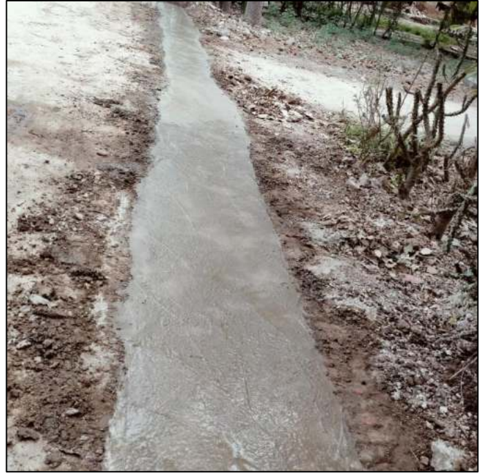
Picture 40: PCC Reinstatement work
