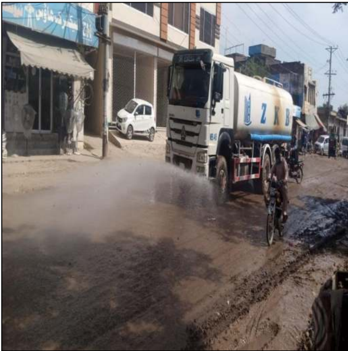
Picture 25: Lot-02: Water Sprinkling at Marala Road
