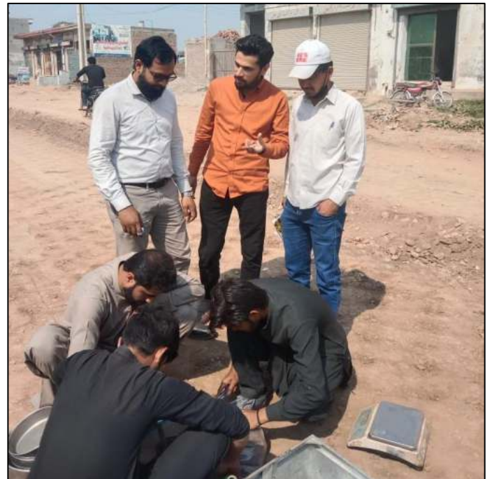
Picture 38: FDT/Sand Replacement testing of Sub Grade Layer at Restoration site
