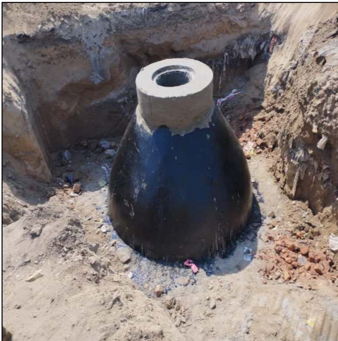
Picture 19: Lot-4 Bitumen costing at exterior of manhole
