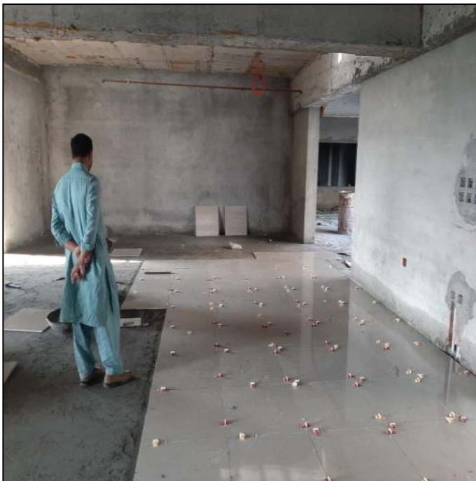
Picture 44: Plumbing work in washrooms at 5th floor
