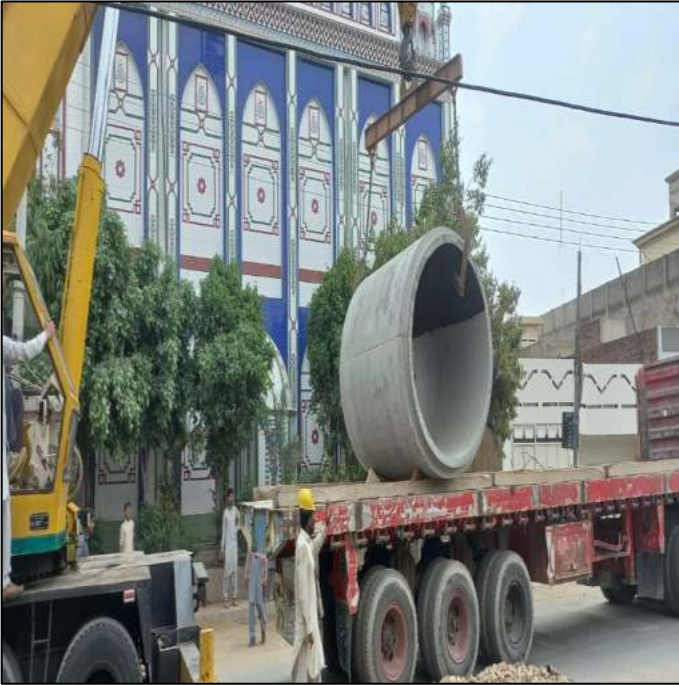
Picture 13: Lot-2 Unloading of Pipes on Madhali Road
