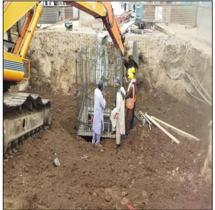
Picture 30: Lot-02: Manhole No. 50 Steel Fixing in progress at Marala Road
