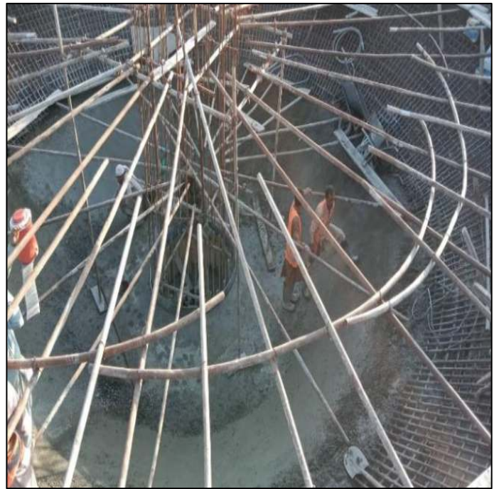
Picture 42: RCC Pouring of OHWT T-40 Bowl
