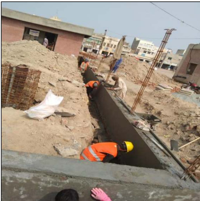
Picture 11: Plaster work on boundary wall at OHR T7 Galla Mandi
