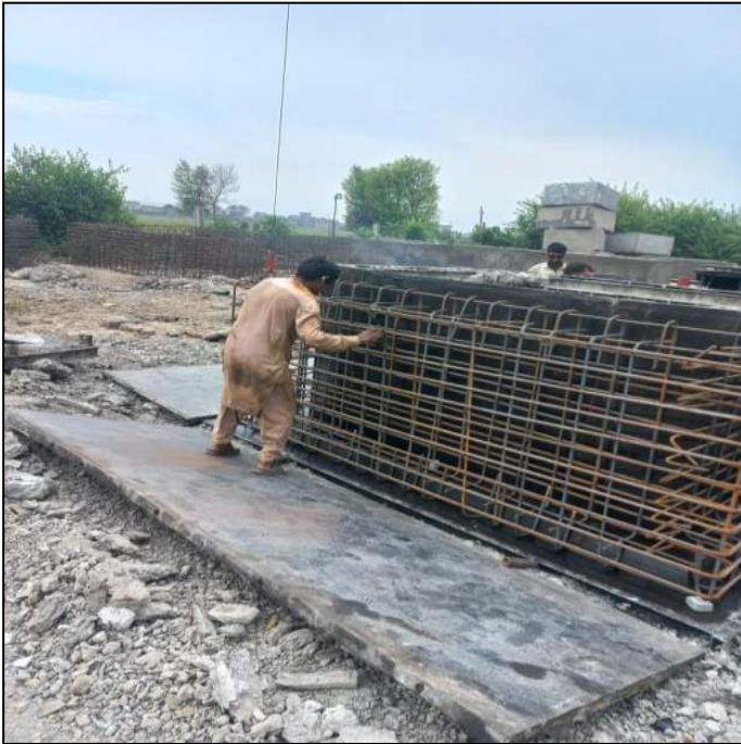
Picture 33: Lot-02: Conduit Steel Fixing in Progress @ Contractor Camp
