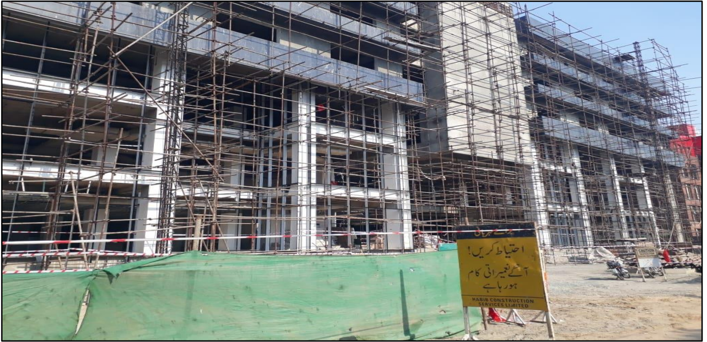
Picture 43: Cladding work on outer walls
