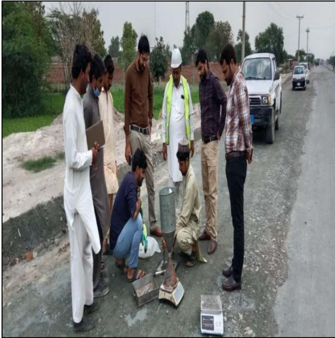
Picture 17: Lot-4 Compaction Test of Water Bound Macadam being conducted
