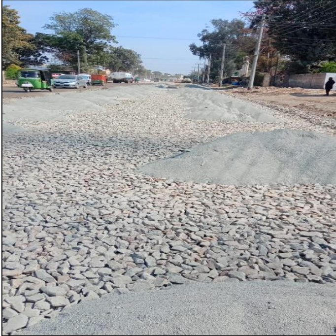
Picture 21: Water Bound Macadam under Construction
