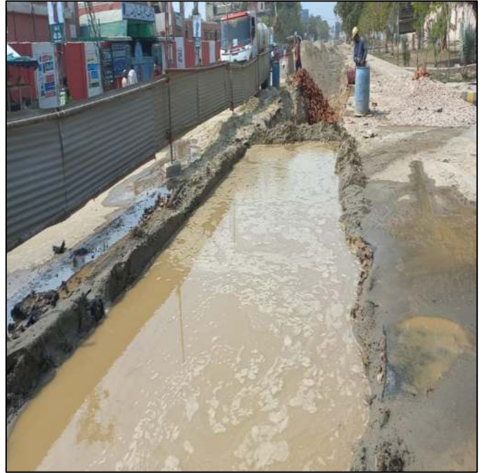
Picture 14: Lot-2 Soil consolidation by water flooding technique
